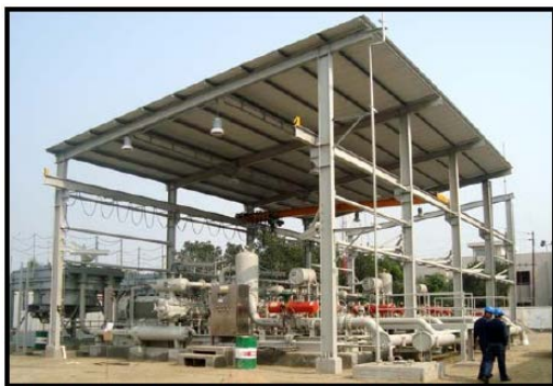
Compressor Project at Mymensingh 210 MW PS – RPCL (Completed and Commissioned in January 2011)
